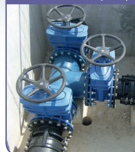
Martigues Power Plant, France, Marseille, AquaGrip
