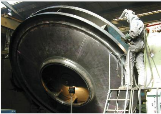
Application of protective paint to a fan unit
