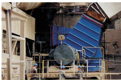
Before and after images showing the revamping of a Kiln ID fan installation
