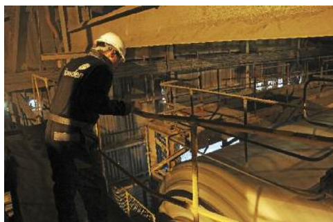
Above: Maintenance inspection at cement plant
