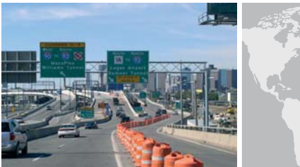
USA (HOWDEN BUFFALO): BOSTON CENTRAL ARTERY TUNNEL
