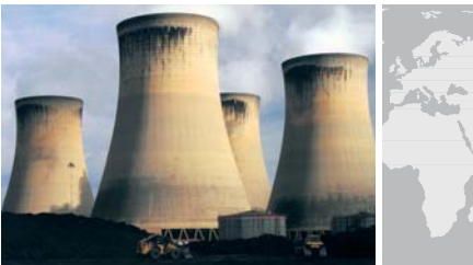
EUROPE: DRAX POWER STATION
